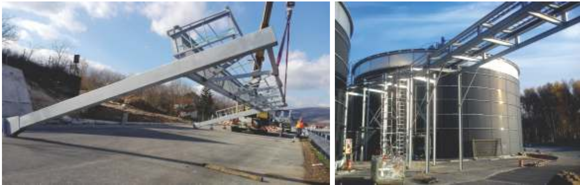
Various hot-dip galvanized steel constructions in acc. to EN1090
