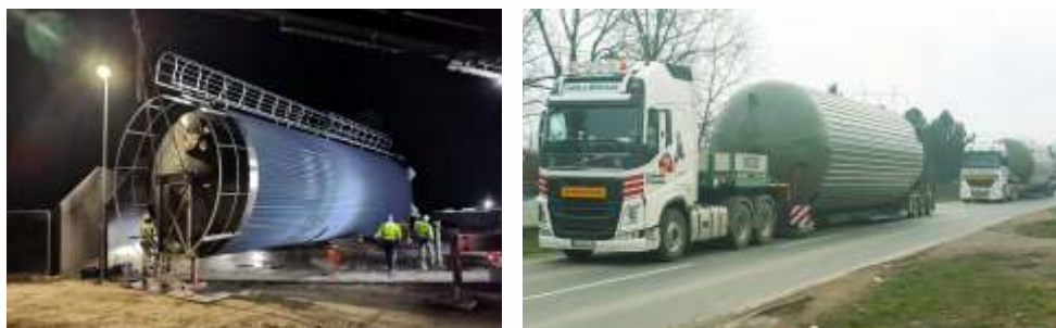
Pic3. Heating tanks up to 6bar and 200m 3
