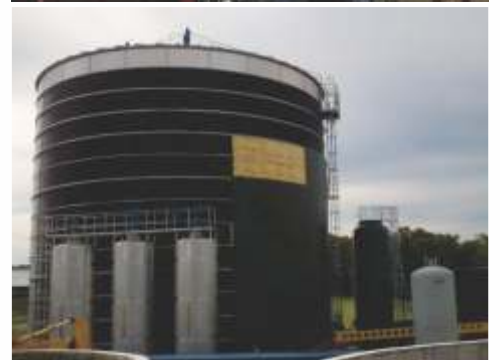
Pasteurization/mixing tanks on various biogas plants (Germany, USA)
