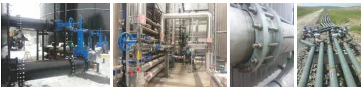
Complete piping packages in carbon and stainless steel (various industrial plants)
